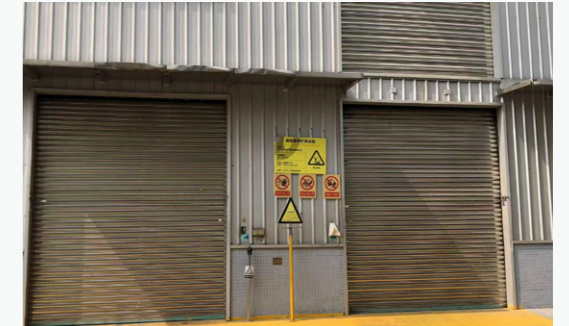
Hazardous Waste Storage Facility
